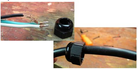
Figure 9. Thread power cord through wire nut.
