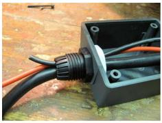
Figure 11. Thread red and black 12" cords through junction box hole.
