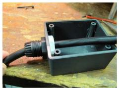
Figure 10. Thread power cord through junction box hole.
